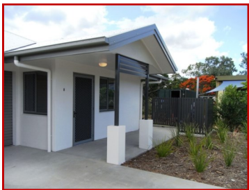
Disability designed units
